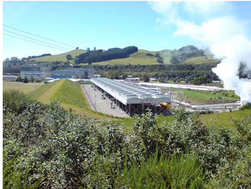
Wairakei Geothermal Plant
