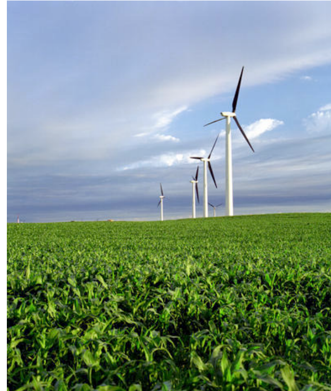
Wind Turbines: Electricity Generator
