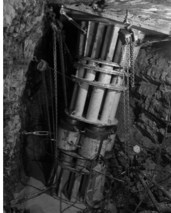
Fig. 2. In-situ plate load test used at Bakhtiary site.
