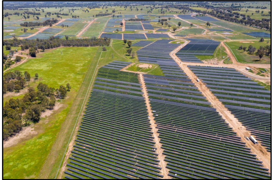
FRV Solar Farm in Queensland
