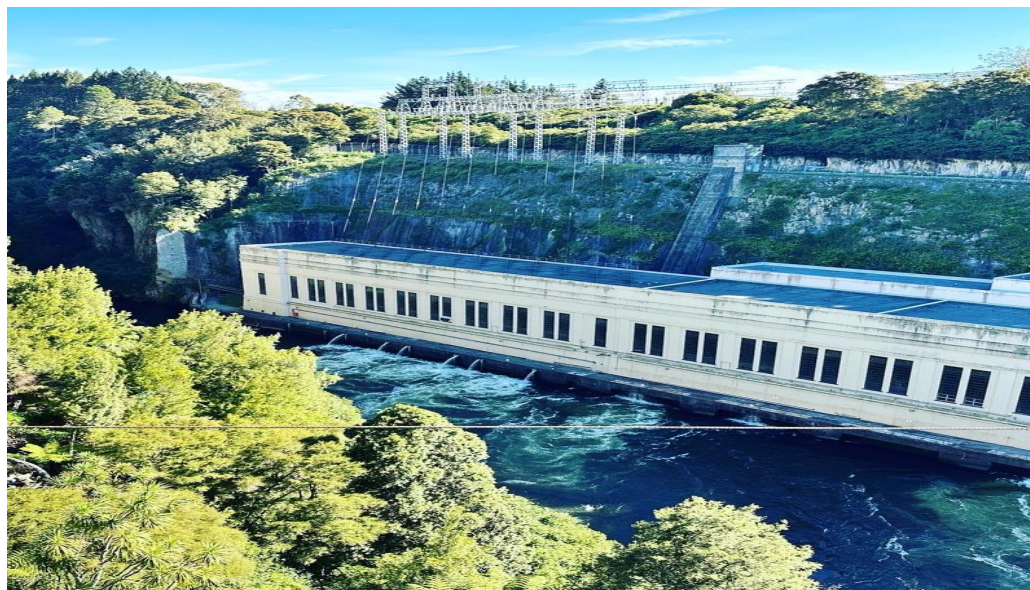
Figure 1: A photograph Captured By Me During Site Visit Of The Arapuni Dam
