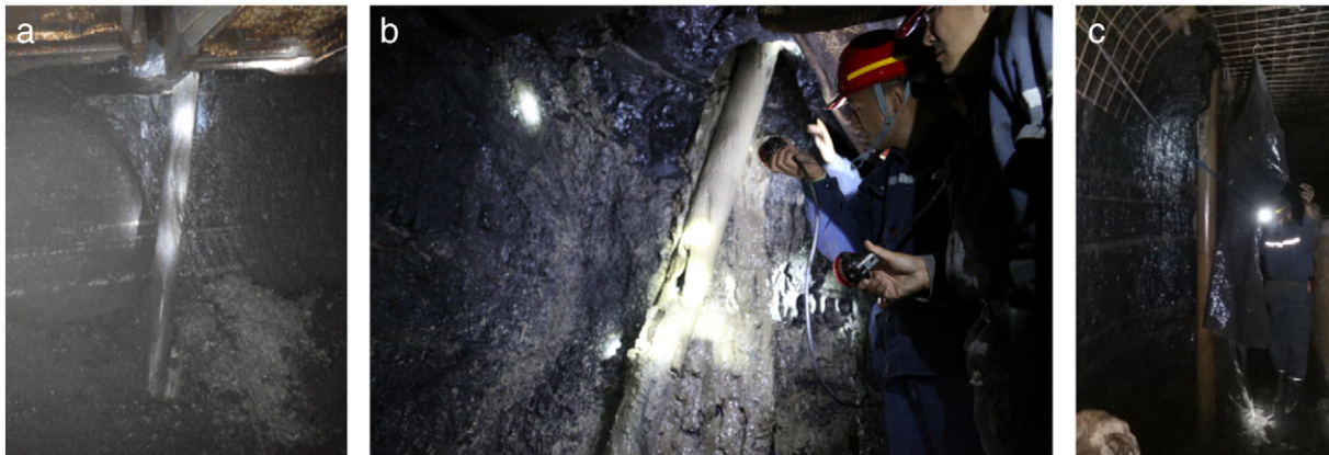
Fig. 1. Images taken underground for three abandoned oil wells exposed at the longwall working face (a, b) and in the gateroad (c) of Hecaogou colliery in the Ordos basin, China.
