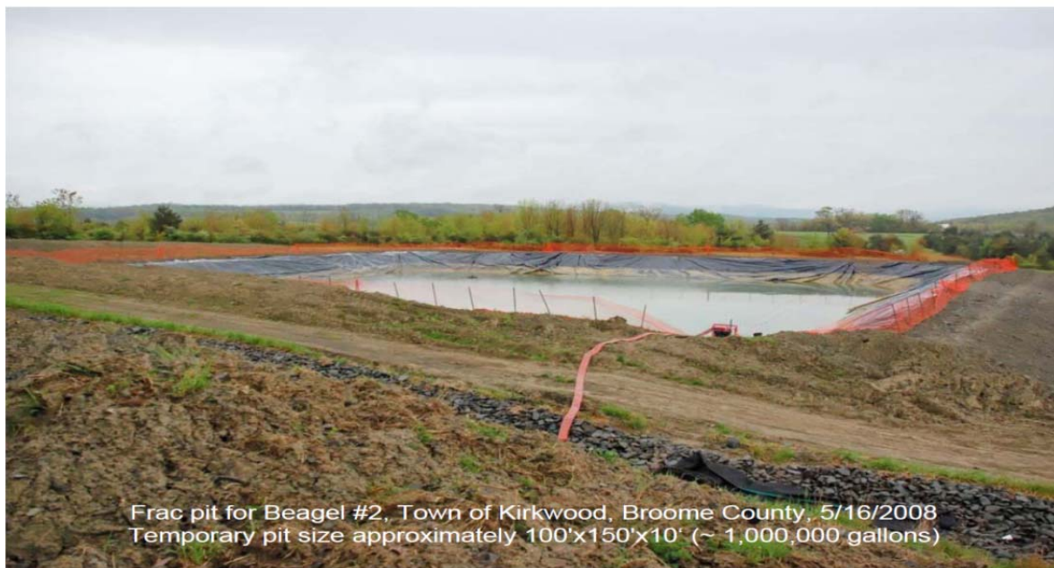
Figure 4.5: A lined storage pit used for storage of water in Broome County NY
