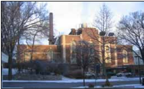
Fig 1. West Campus Steam Plant
