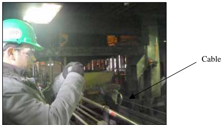
Fig 23. Coal Loading mechanism at WCSP
