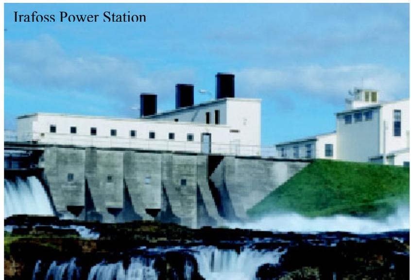
Reykjavik. The Irafoss station harnesses power from two falls, the Irafoss and Kistufuss, located on the lower Sog. The combined head of the two falls is 38 meters. When it went online in 1953 it utilized 2 turbines that each generated 15.5 MW. In 1963 an expansion of the plant added a third turbine, which has a generating capacity of 16.7 MW. Interestingly, one of the brands of generators they use is Westinghouse Electric, International Co. of the United States.
