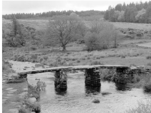
Figure 15: Clapper Bridge, Postbridge, Dartmoor, Devon. Photo by M. Pickett, May 2003.
