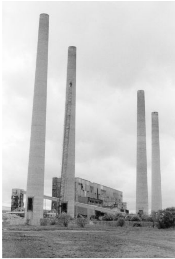
Figure 5: Abandoned power plant. Photo by M. Pickett, May 2003.
