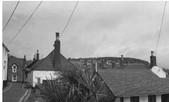
Figure 24: Electricity infrastructure is easily ignored by those accustomed to it. Photo by K. Johnson, May 2003.
