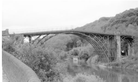
Figure 19: Iron Bridge. Photo by M. Pickett, May 2003.
